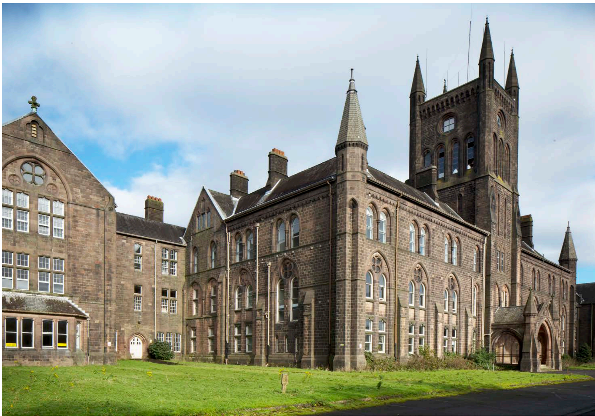
LANCASTER MOOR HOSPITAL, LANCASTER (BEFORE)
