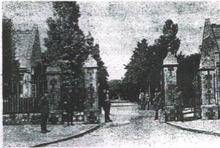
Hospital Gates during the American occupation, 1918.
